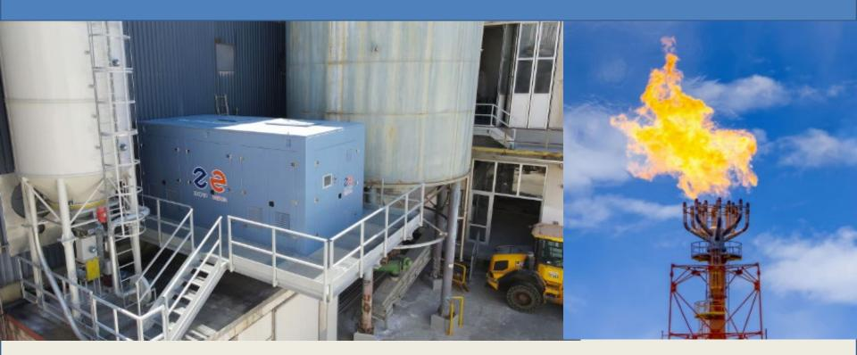
MR partner Zuccato Energy designs and manufactures ORC (Organic Rankine Cycle) systems to transform the heat generated by industrial processes, gas flaring, motors and renewable sources into clean electricity with high efficiency.
